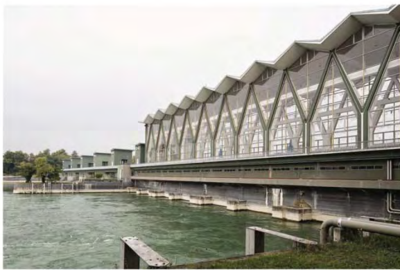
17 Kraftwerk Birsfelden, Switzerland, 1951, Hans Hofmann
