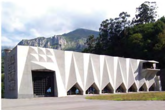
18 Hydroelectric Plant Proaza, Spain, 1968, Joaquin Vaquero Palacios
